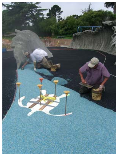
Resilient play surfacing installation in wave wall areas showing sea turtle sculpture location (View northwest)
